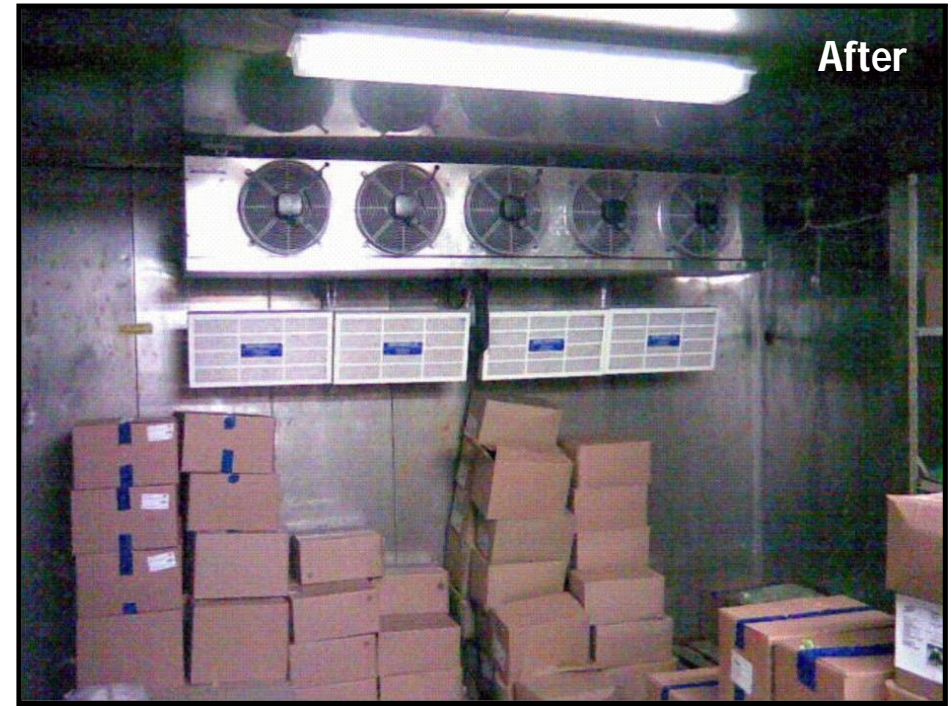
Refrigerated food storage area before and after CoolSaver Catalytic Panels are installed to dehumidify and remove icing from the chill room area
